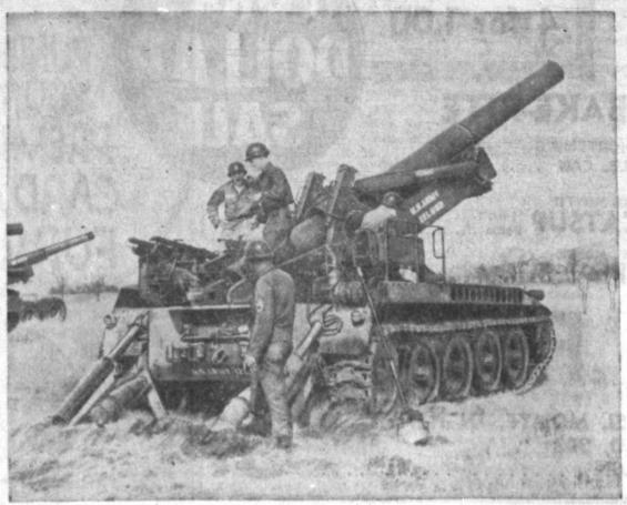
ARSENAL NEWCOMER — Crew of a new U. S. Army M-110 eight-inch howitzer prepare it for firing at Renton, Wash. The hydraulically-operated spade at the rear of the self-propelled vehicle anchors the field artillery piece against the recoil.
