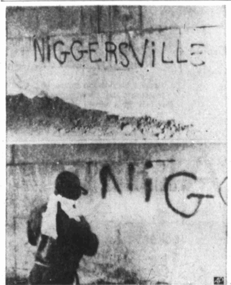
Vandals' Slur A workman removes a racial slur painted in pink letters on the wall of an underpass beneath Memorial Bridge near the Lincoln Memorial in Washington, apparently a day after the 100th anniversary of the emancipation proclamation celebration. Another slur, "nigger lover", was painted on a rear wall of Lincoln memorial. These films made available from CBS News film.
