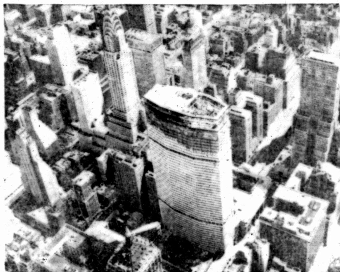
SKYLINE NEWCOMER — You're looking down at the nearly completed 59-story Pan American World Airways building at 44th Street and Park Avenue in New York. It's built over tracks of New York Central and towers over Grand Central Terminal.
