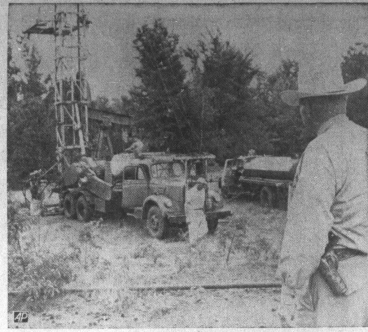
Texas Ranger R. L. Badgett stands watch as crew begins testing oil well near Greggton for deviation. The Texas Railroad Commission is in process of testing several wells in the rich East Texas field for crooked drilling.
