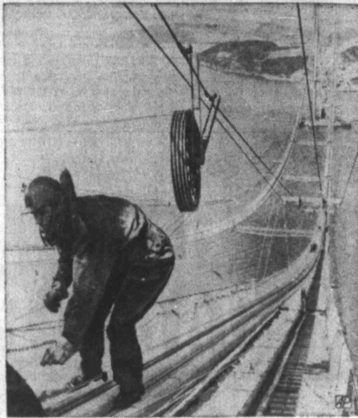
HIGH WIRE MAN — A workman inches up catwalk of Scotland's Forth Road bridge which will be Europe's longest suspension bridge when completed in 1963.
