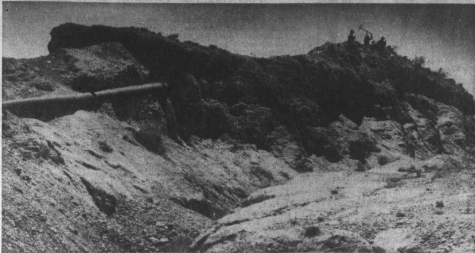
Pipe To Be Moved—Ridge To Disappear
