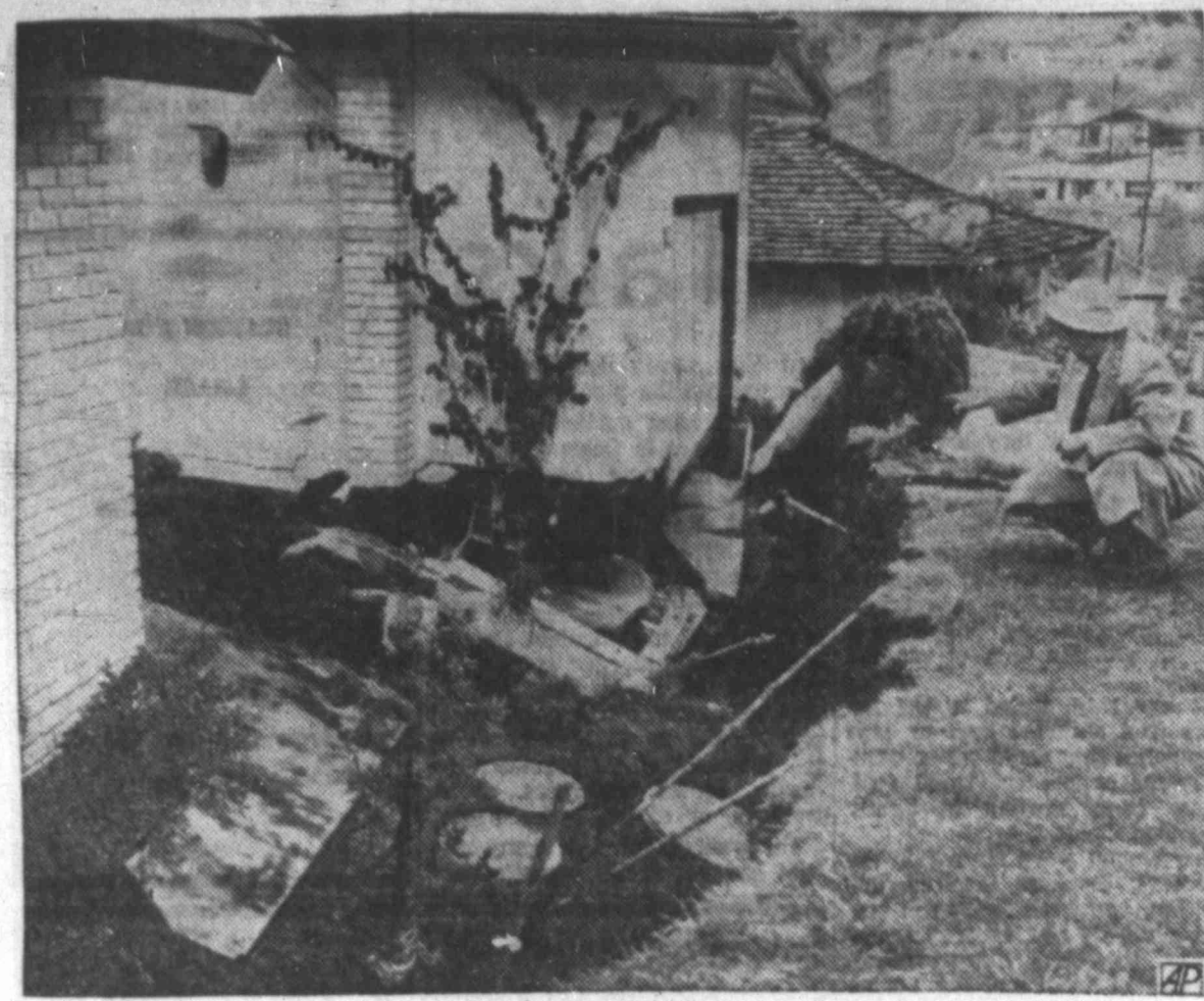
Damaged By Storms
