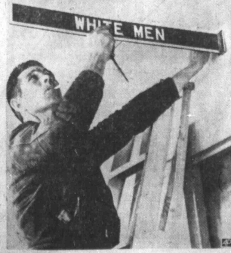
Signs Come Down A workman removes a rest room sign at Montgomery, Ala., Municipal Airport in compliance with a federal court order banning segregation. However, city officials delayed plans to remove waiting room furniture and other facilities and said the airport restaurant will be closed if there is a concerted integration attempt.
