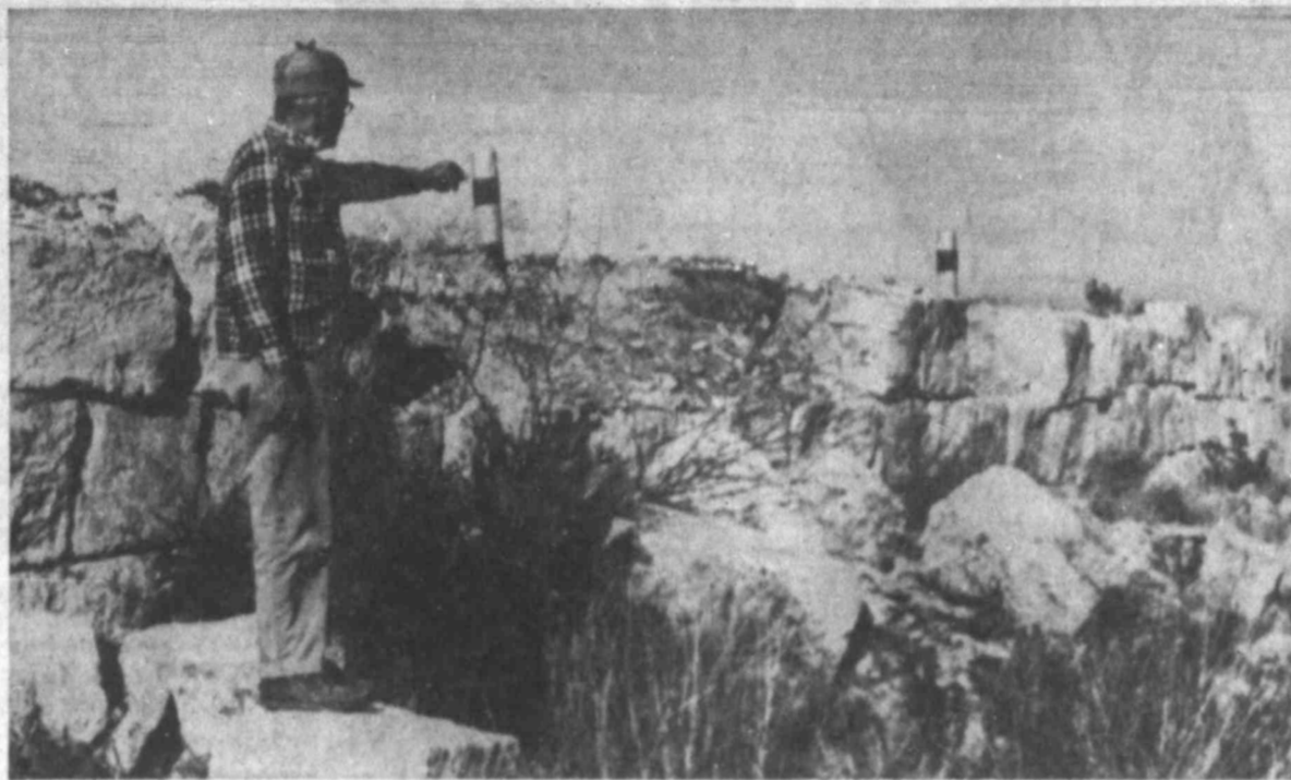
ROAD BED LOSES ROCK SUPPORT A. B. Cramer points out vandalism
