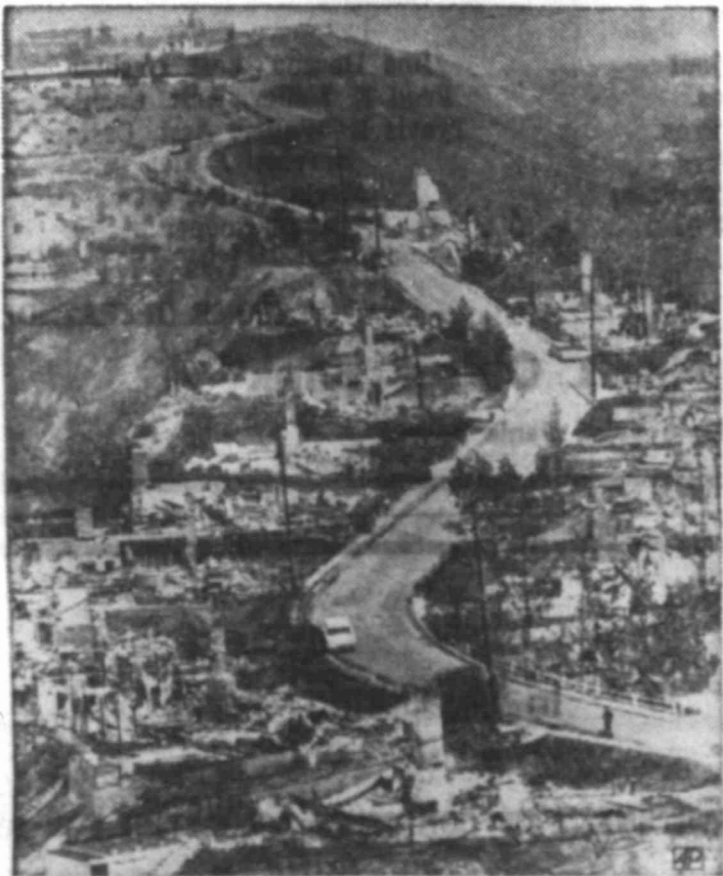
FIRE WAKE —Homes lie in ruins on Linda Flora Drive in Bel-Air section of Los Angeles following November brush fire. It was the worst fire in the city's history.
