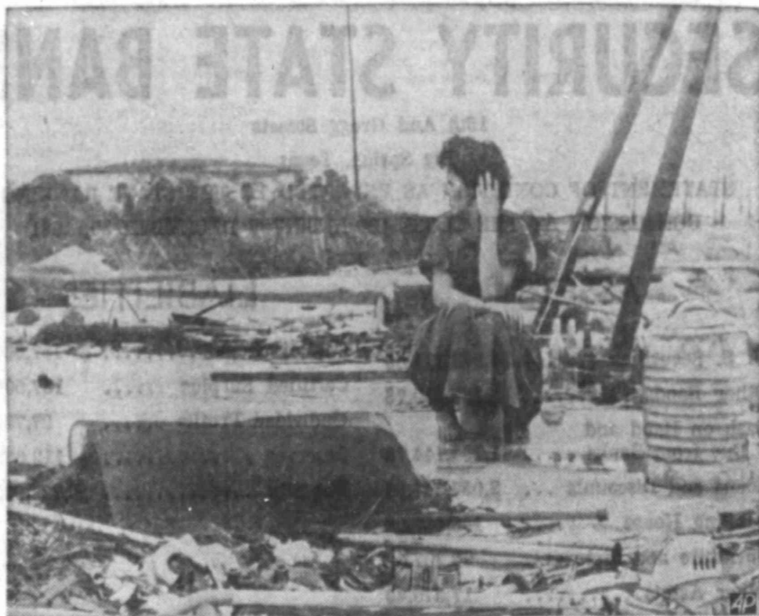
AFTER FURY PASSED —Mrs. Joy Evans, dazed by destruction of Hurricane Carla, sits on foundation of what was her home in Port O'Connor, Tex. The September storm, sweeping inland from the Gulf of Mexico, caused heavy damage in the Southwest.
