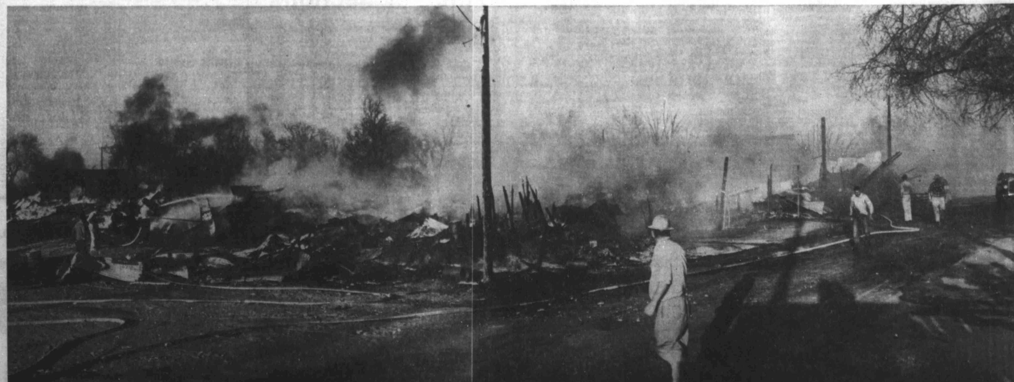
A quarter of a city block was left in ruins when Coahoma's Burton-Lingo Lumber Co. buildings burned Thursday
