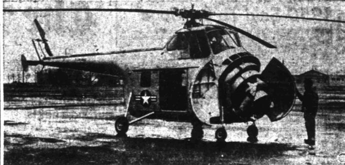
Clam-shell doors swing open to show the engine of the new H-19 Sikorsky helicopter just flight-tested successfully by the Air Force at Bridgeport, Conn. Transfer of motor from behind pilot to the 'copter's nose gives more passenger and cargo room to the craft, which was designed for search, rescue and liaison work. The H-19 can carry eight litters and one attendant, or 10 passengers.
