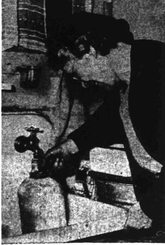
New Yorkers may be fretting about the water shortage, but it doesn't worry the ingenious Brooklynites who live in the Kiendleville section. They take rain water directly from their roofs. Picture shows the gimmick—a rain pipe leading down from the roof to a big storage drum. From the drum a hose goes into the house and connects up with the kitchen faucet. Mrs. Wilhelmina Peppers, center, is seen drawing a gallon of rain water-and laughing at New York's water shortage.
