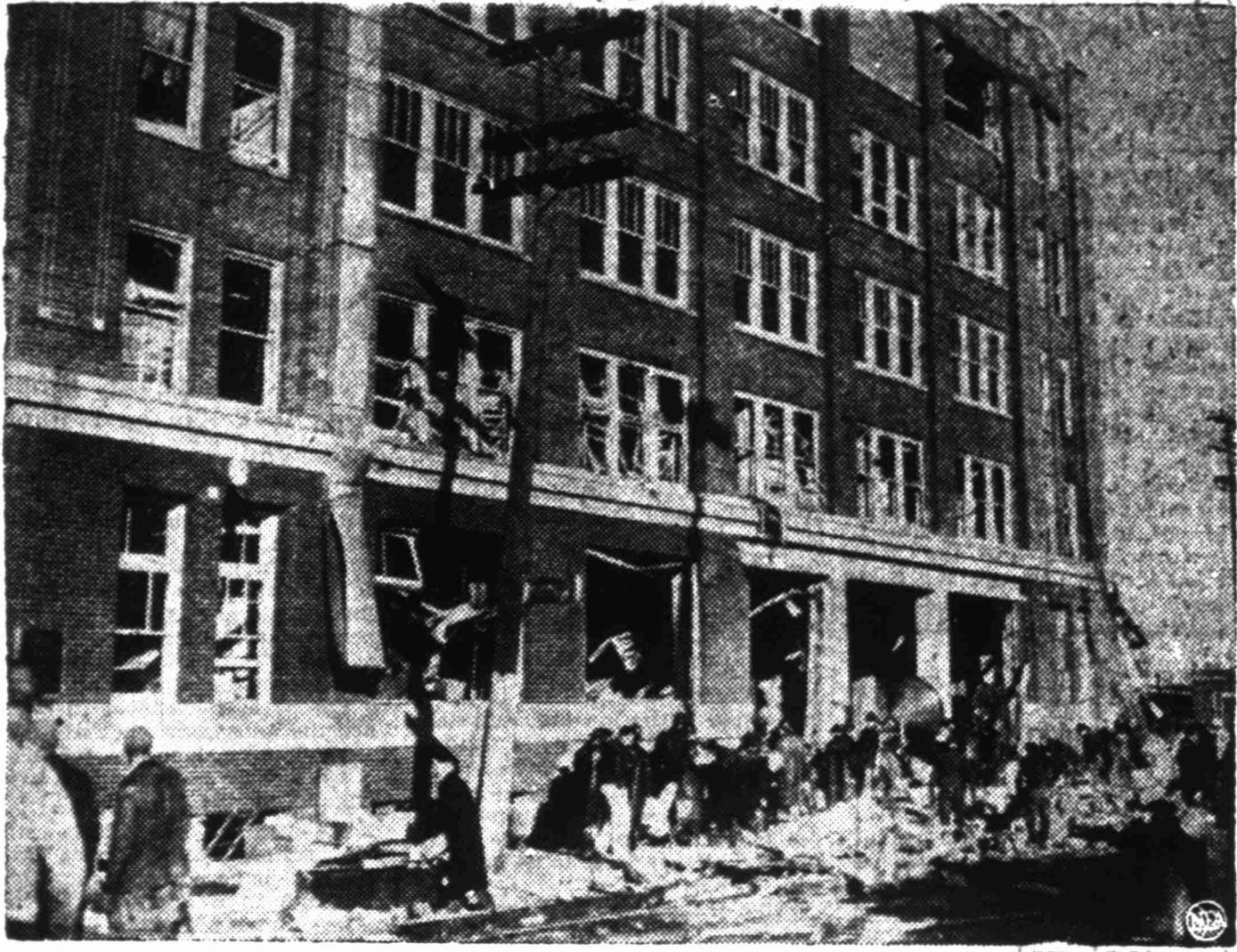
This was the general scene of destruction at the Swift & Company office building in Sioux City, Iowa, following a disastrous explosion. Sixteen were killed and more than 80 were injured.
