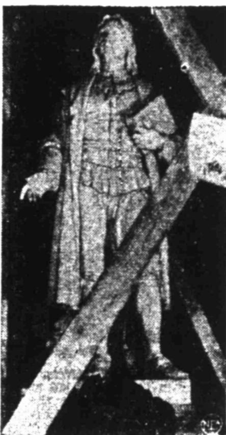
Statue of John Adams stands among scaffolds in Statuary Hall.
