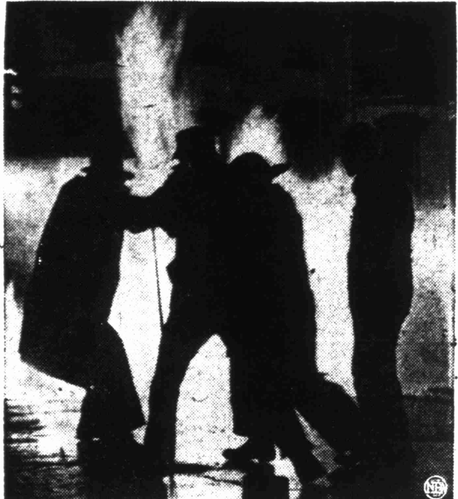
(NEA Telephoto) Damage estimated as $100,000 resulted from fire and flood in Allentown, Pa., when an exploding gas main blew up a large water main in the heart of the city. Here, workmen, silhouetted against the flames, attempt to turn off the valve of gas main.
