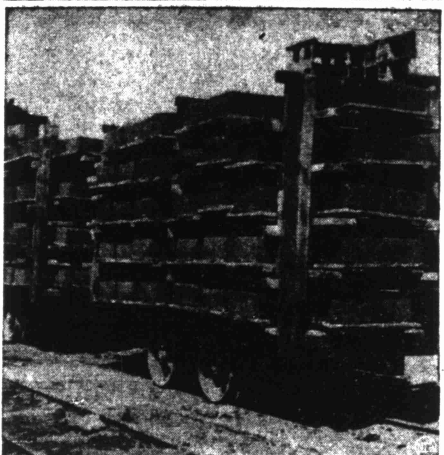
War ruins in Warsaw, Poland, are providing the bricks badly needed for reconstruction. In special mills located near the devastated areas rubble is ground, sorted, mixed into concrete and finally pressed into bricks. Above, workmen move the ground rubble toward the concrete mixers. Below, the finished bricks are hauled on lorries to construction sites.
