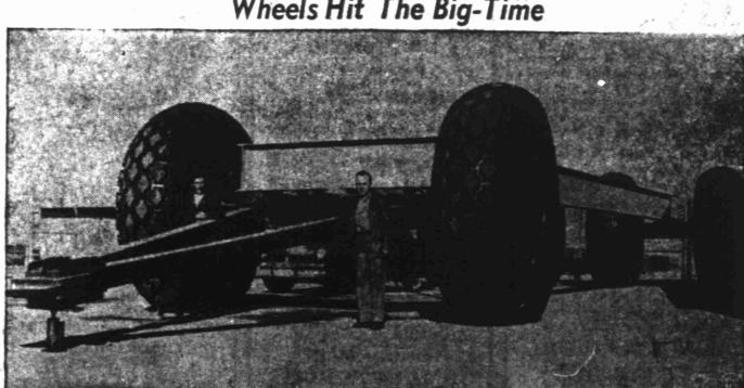
Dwarfing two men and the automobile in the background, this huge four-wheeled trailer, pictured in Akron, Ohio, will carry oil derricks in the Arabian oil fields. The tires are the largest ever to be built con mercially. Each one is almost 10 feet in diameter, weighs more than 3,500 pounds, and carries a 55,000 pounds.
