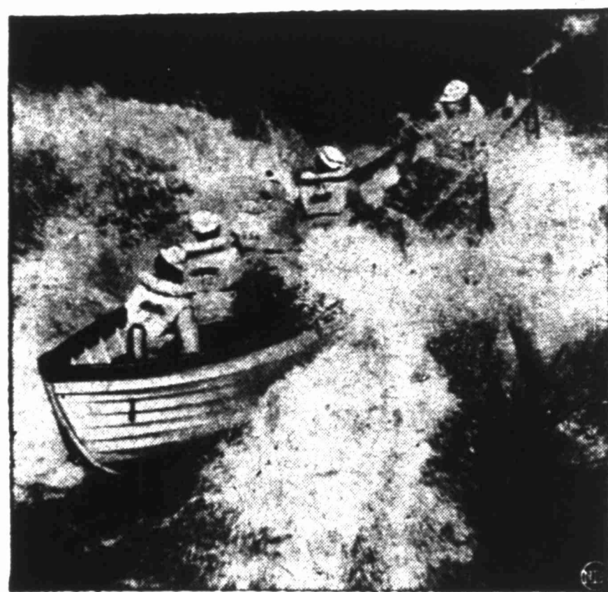
The conventional method of lowering a lifeboat on long ropes from davits over the side of a ship, in use for hundreds of years, requires several men and up to two minutes in time. But the U. S. Coast Guard has come up with a new idea, called the "Pease Cradle," that does the job in five seconds and with only one man at the engine to work the cable, left. The cradle lowers a loaded boat to the water with a huge splash five seconds later, above. The method, which is expected to revolutionize sea rescues, is being tested at the Coast Guard Research and Development Division at Curtis Bay, Md.
