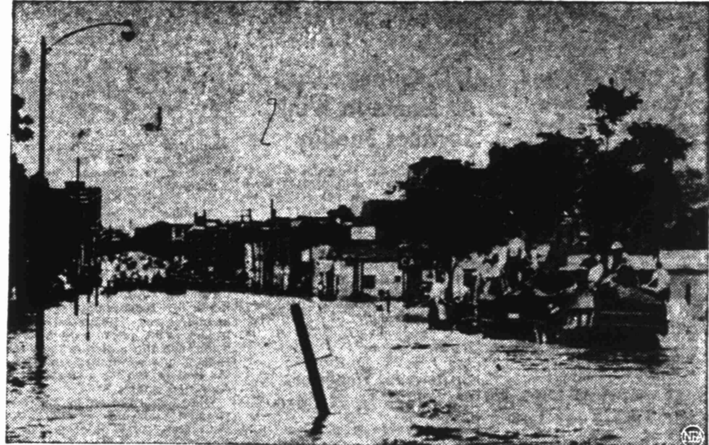
Two trucks, at right, filled with sand and pulled by a tractor, head toward a crowd of townfolk, in distance, who are forming a human chain across one of Dodge City, Kansas', principal streets as they fill sand bags in an effort to keep back waters of the overflowing Arkansas River.
