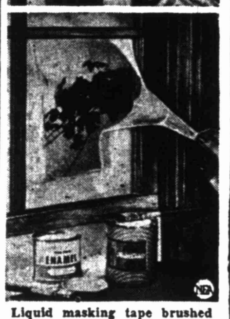
Liquid masking tape brushed on window panes (top) protects glass from paint splatters. When painting is finished, tape peels off easily (bottom).
