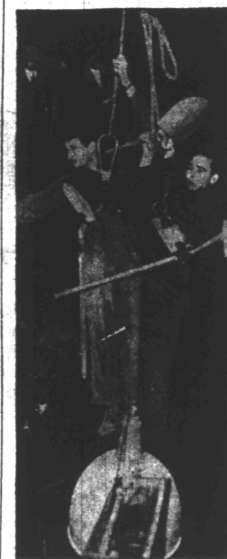
(NEA Telephoto) Two workmen are lowered into an excavation dug beside a 120-foot well shaft in San Marino, Calif., in a futile attempt to rescue three-year-old Kathy Fiscus, trapped 100 feet below the surface of the earth. Albert Linnel, right, and John Inhart, left, drove a lateral shaft from the bottom of the excavation to the rusty, 14-inch casing through treacherous, sandy soil.
