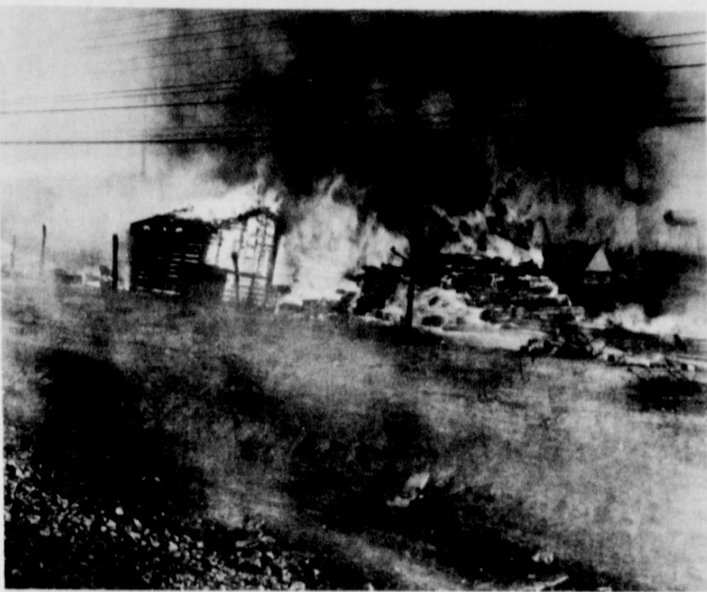
FEEDLOT FIRE —Property of the Wells Brothers just east of Friona was hit by fire Monday afternoon of this week during the height of the high winds which raked the area. Some wooden corrals and a small shed
