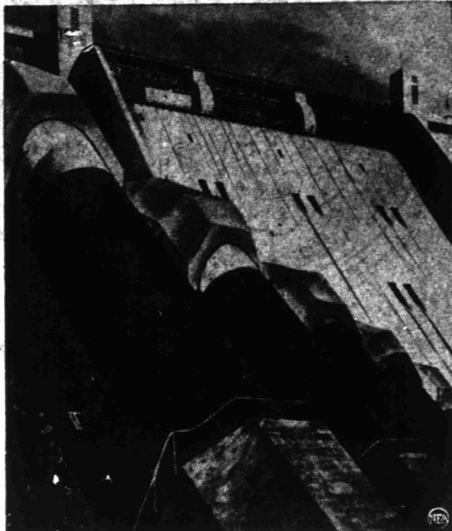
This is one of the mighty Shasta Reservoir penstocks, ready to feed water to the turbines in California's Central Valley power project. Although power isn't being produced, it has already generated a major controversy.
