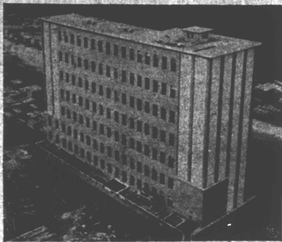
American funds are doing a big job in Europe, and here's a concrete example. This flour mill in Trieste was almost completely destroyed during the war, but U. S. aid funds rebuilt it into the largest and most modern plant of its kind in the Mediterranean area. It's now handling Marshall Plan flour for Trieste and Austria, and its silos hold 30,000 tons of grain.
