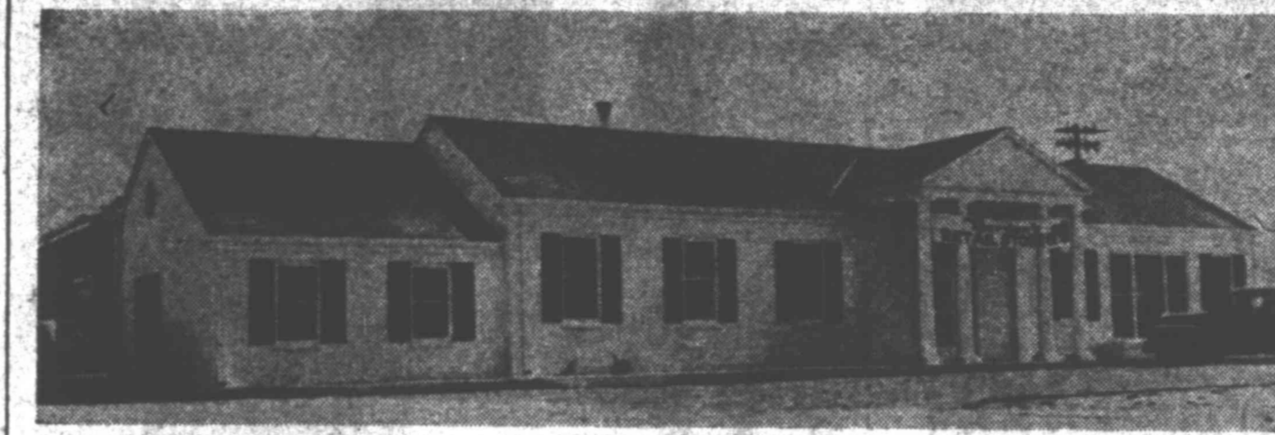
Open house will be observed Sunday afternoon at the new and completely modern plant of The Borden Company at the intersection of West Missouri Street and U. S. 80 Highway in Midland. The plant was completed recently at a cost of more than $300,000.
