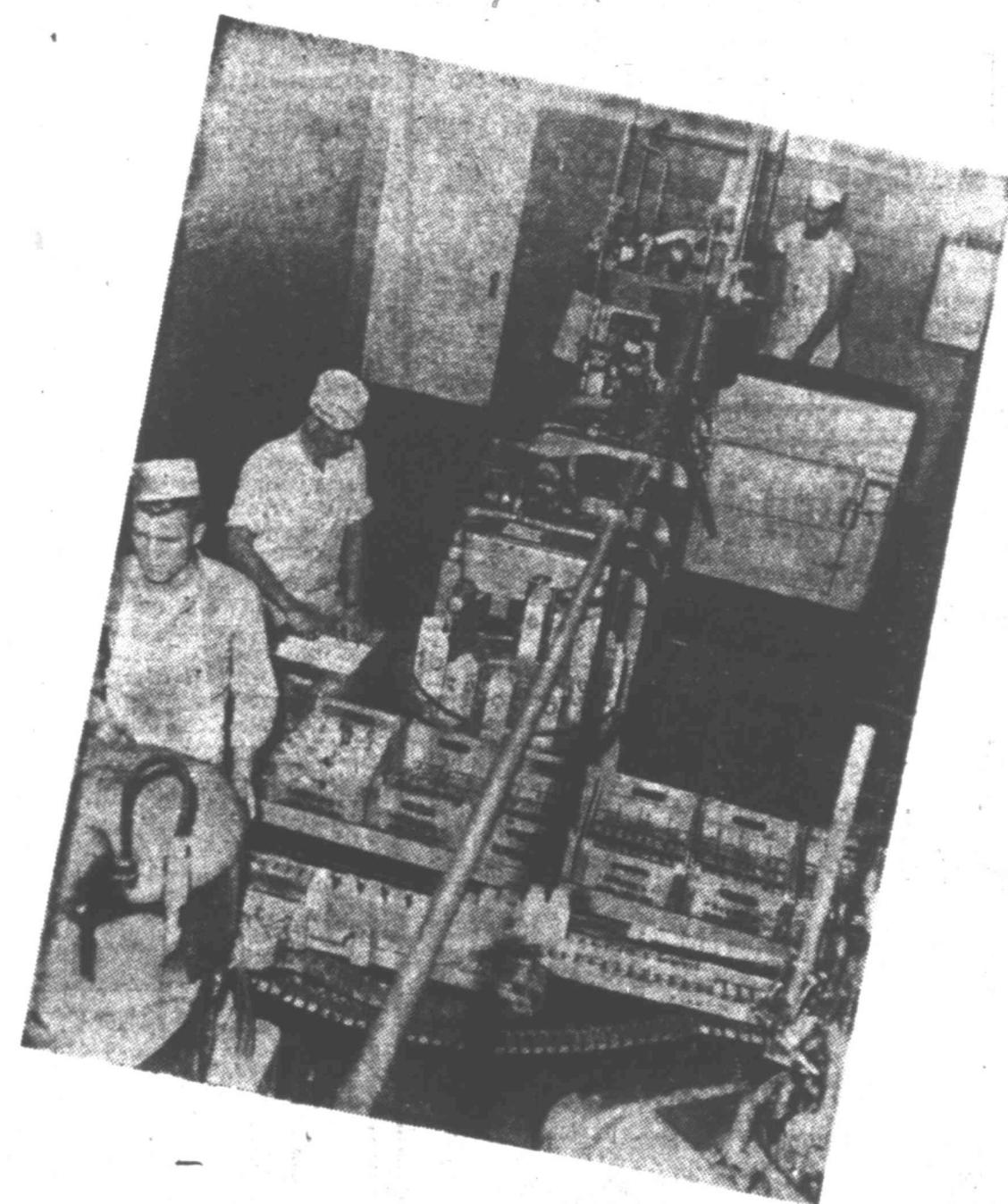
The above Pure-Pak machine automatically fills sterilized paper cartons with Borden's homogenized milk and then seals them with a wax coating with a capacity of 35 quarts per minute.
