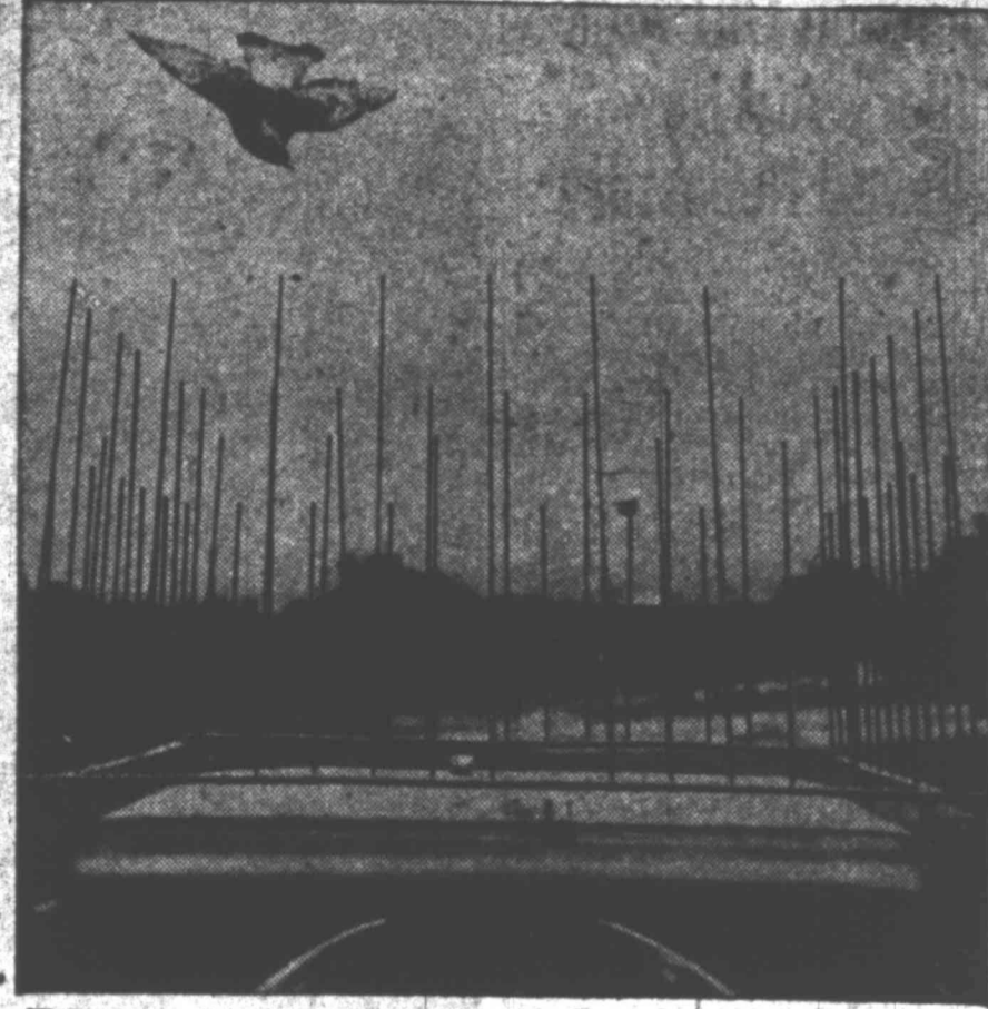
This pigeon at Cleveland Municipal Airport is a bit flustered by the pronged device which keeps him from roosting atop the fog landing light. That's what engineers of the Westinghouse Electric Corporation had in mind when they designed the gadget to keep birds from obscuring the face of the lamps and creating a hazard for incoming planes.
