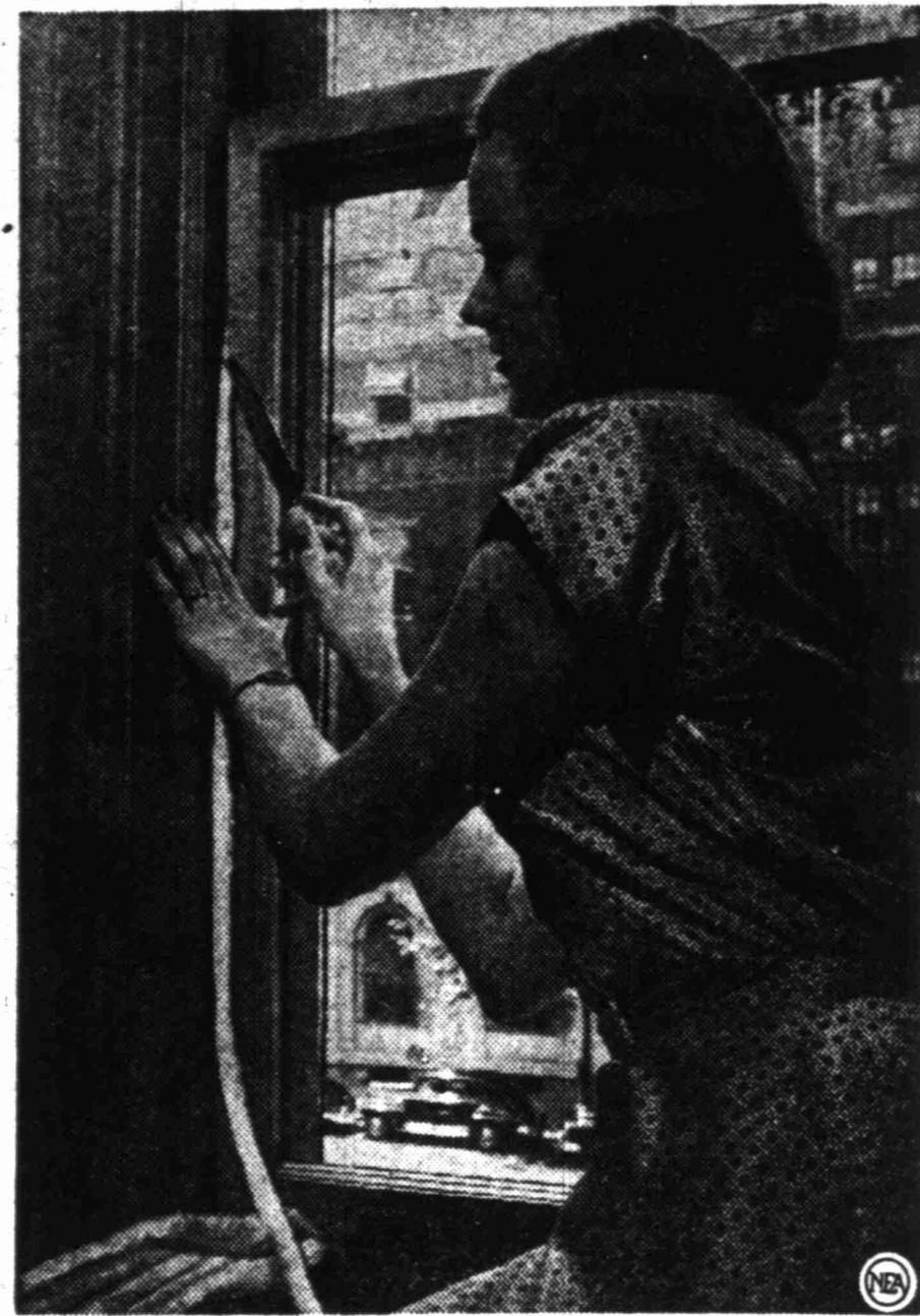
Soft, pliable rope of glass fibers makes this new weather-stripping. Young housewife seals up window crack by poking strip in place with a kitchen knife.
