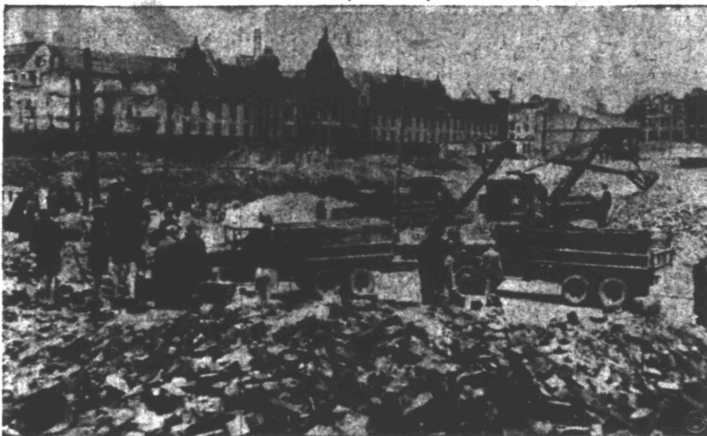
The U. S. Army is rushing new air facilities in Berlin, to relieve the city's overtaxed airfields. Cranes and bulldozers load trucks with the rubble of buildings bombed and blasted during World War II. The rubble is used as a base for a new air strip at Tempelhof Field. (Photo by NEA-Acme staff correspondent Al Cocking)
