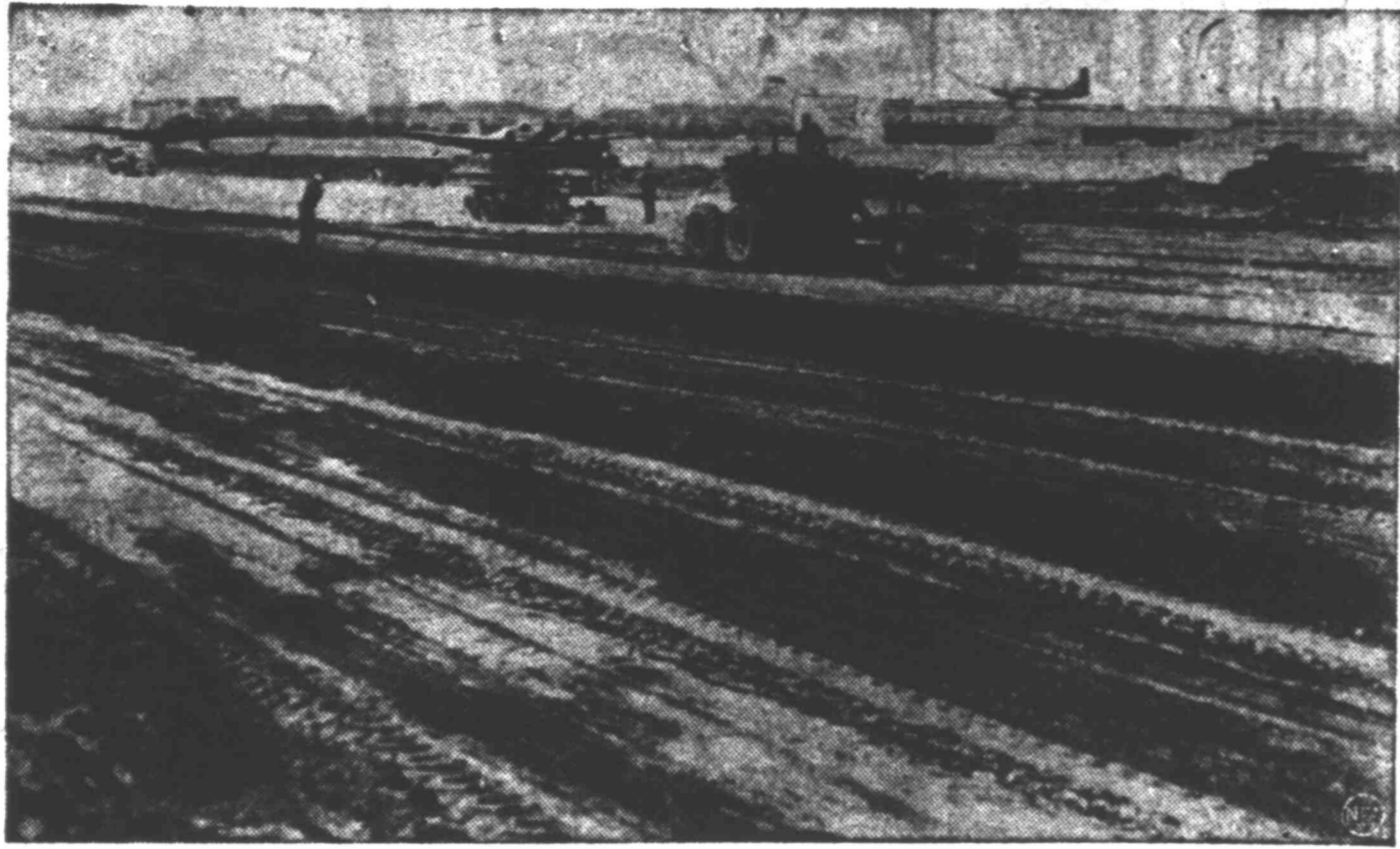
Since the Russians clamped down their blockade on Berlin, the U. S. Army has been flying food and other supplies to the beleaguered people of Berlin. The greatly increased air traffic has overcrowded the city's airfields and the Army is rushing emergency facilities. Here, Army equipment levels an emergency strip at Tempelhof airfield, built over a base of war rubble. (Photo by NEA-Temple staff correspondent Al Cocking.)
