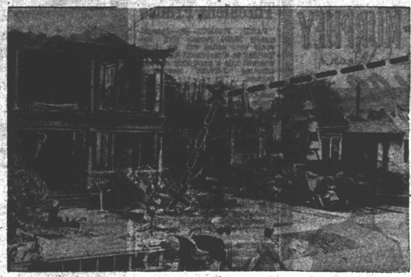
This is a general view of three frame dwellings near downtown San Antonio, Texas, after they were gutted by fire. An AT-3 type aircraft crashed into the center house killing a woman at (X), then fell against the house at left, setting it afire.
