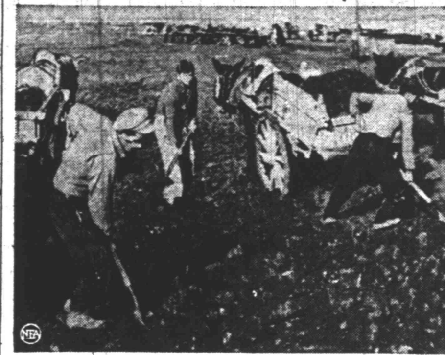
Before U. S. aid came along, "prime movers" in the job of road-building in Greece were a man, a shovel, and a donkey cart. Now U. S. construction men have stirred up an industrial revolution as Greek road-builders discover machines.
