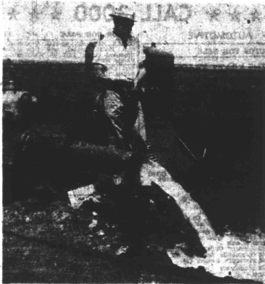
A 1,100 gallon per minute water well has been completed on the Midland County farm of Mr. and Mrs. Charles R. Hall about three miles south of Wrenfield. It is one of the area's largest. The well, the seventh drilled by Hall in search for water for irrigation purposes, is 109 feet in depth. He plans to irrigate about 150 acres of his farm. Leroy Hall, son of Mr. and Mrs. Hall, is pictured watching the flow of water from the big well.
