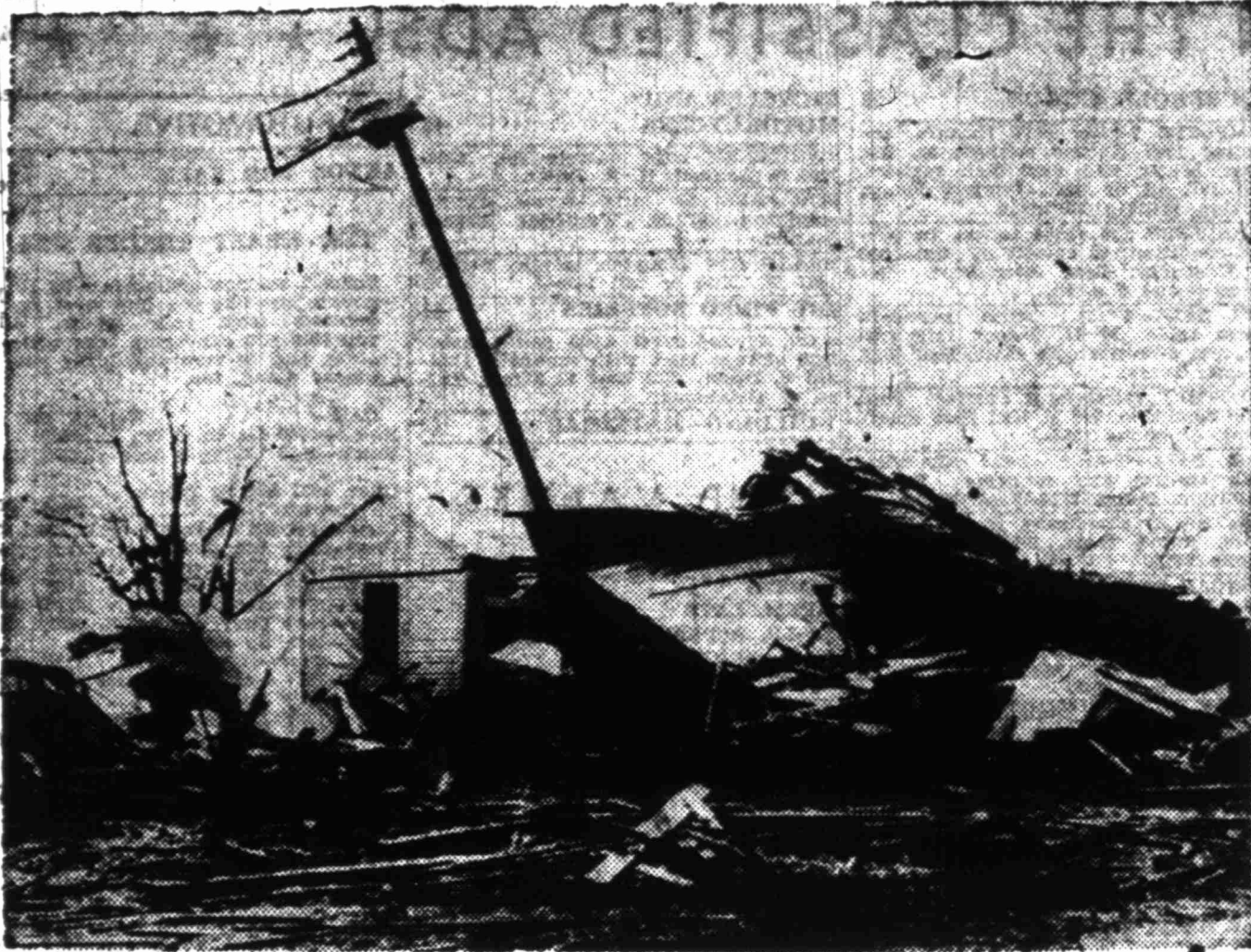
The beginning of the tornado which swept through four states did considerable damage in Southern Missouri. Here on Route 50 near Jeffersburg, Mo., this farm house was demolished. Note the sheets of steel wrapped around the tree and telephone pole.
