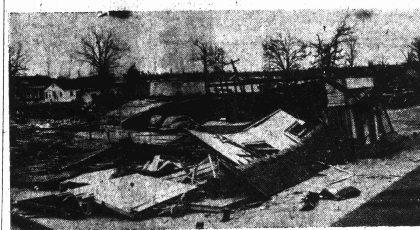
Damage to the business section of Cotton Valley, La., is graphically pictured in this photo, which was made after the tornado passed. In the foreground is what was once the railroad depot and at left background is the scattered wreckage of the C. W. Campbell store.
