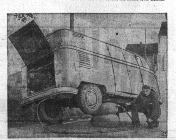
HE SAYS IT'S EASY - Wilhelm Ochs of Kassel, West Germany, shows how he changes tires. He makes a pneumatic jack by using balloon tires inflated by car's exhaust gases. A metal plate is placed between balloon tires and the vehicle's underside.
