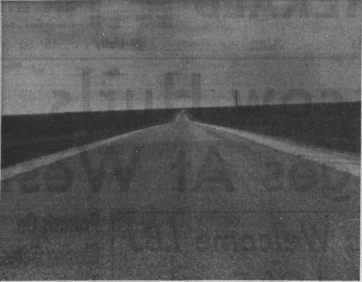
New Hartwells Road Opened
