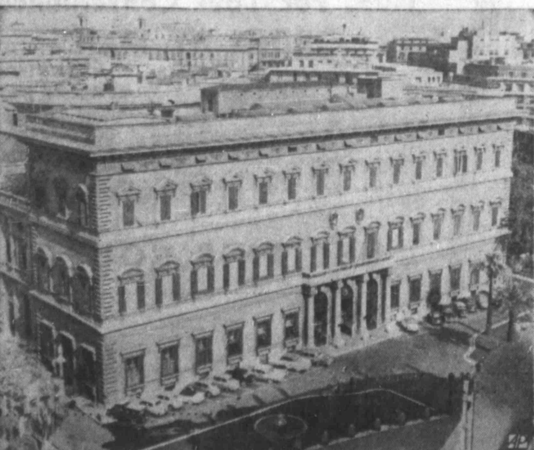
U. S. EMBASSY IN ROME — This is the main building of the United States Embassy in Rome. The building, purchased by U. S. government in 1946, is located on Italian capital's fashionable street, Via Veneto, in one of the city's highest quarters.
