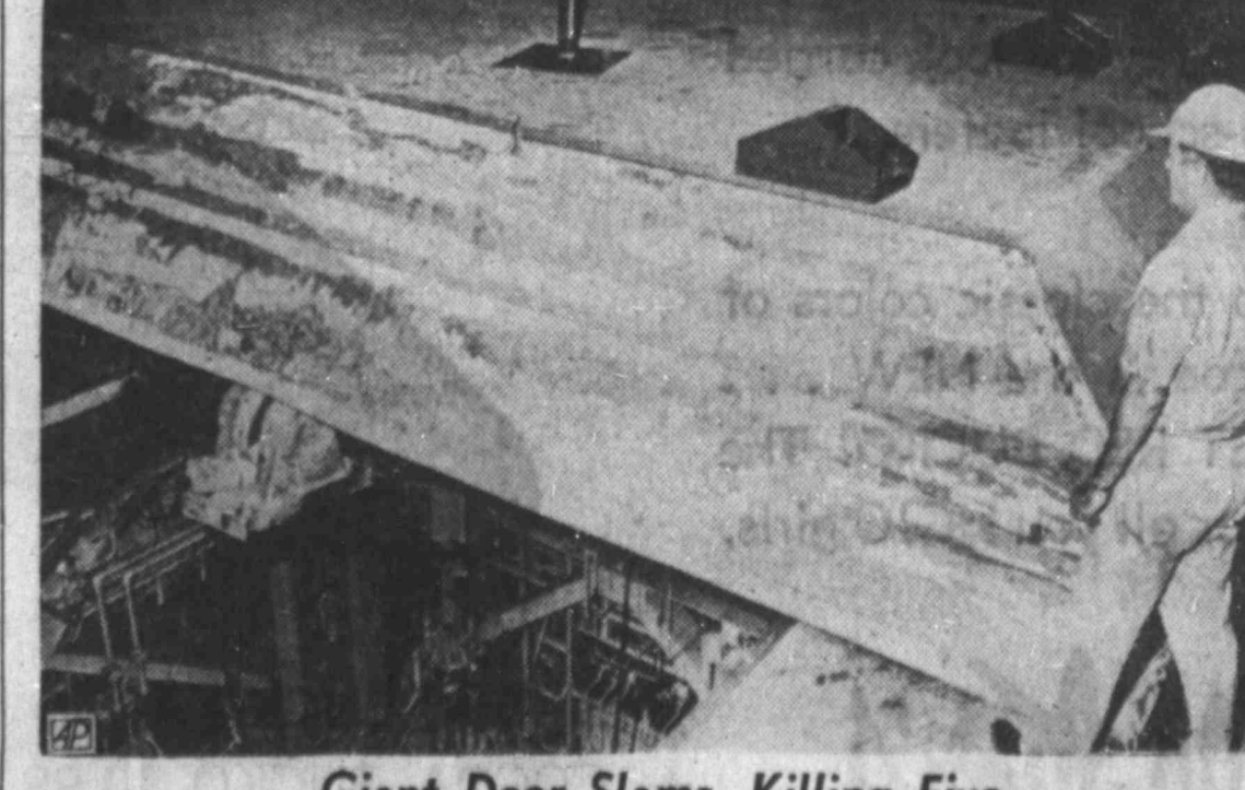
Giant Door Slams, Killing Five This 35-ton steel and concrete door atop a Titan missile launching site near Denver, Colo., slammed shut, killing five workmen and injuring eight others. The massive door is one of a pair which are raised hydraulically as a missile rises to the surface. A spokesman said either a hydraulic failure or failure of a retaining cable caused the door to crash. Lt. Col. William E. Martin, an Air Force public relations officer, stands beside the door.
