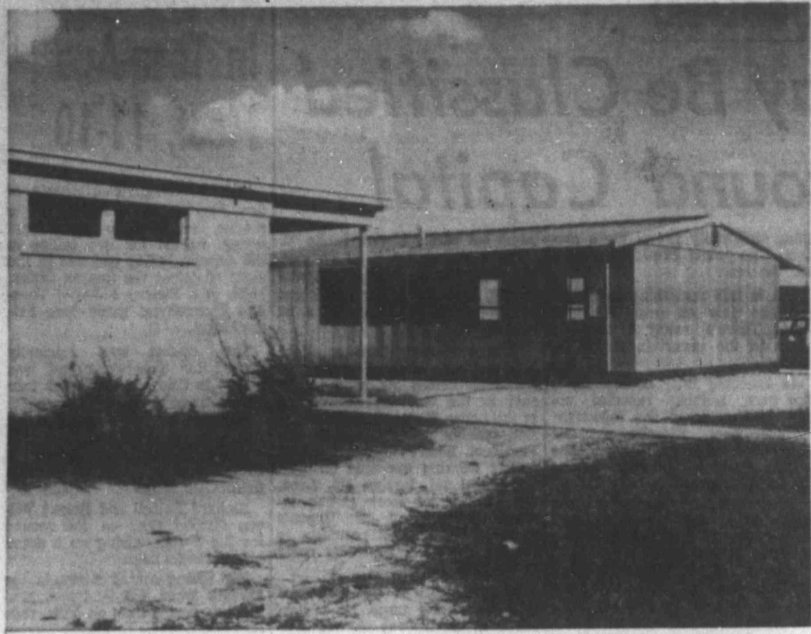
Four elementary schools picked up new classrooms during the summer. They are portable classrooms which can be moved to other schools, if enrollment dips where they are now and increases at another school. This one is at Washington Place Elementary. Others are at Bauer, Airport and Cedar Crest.
