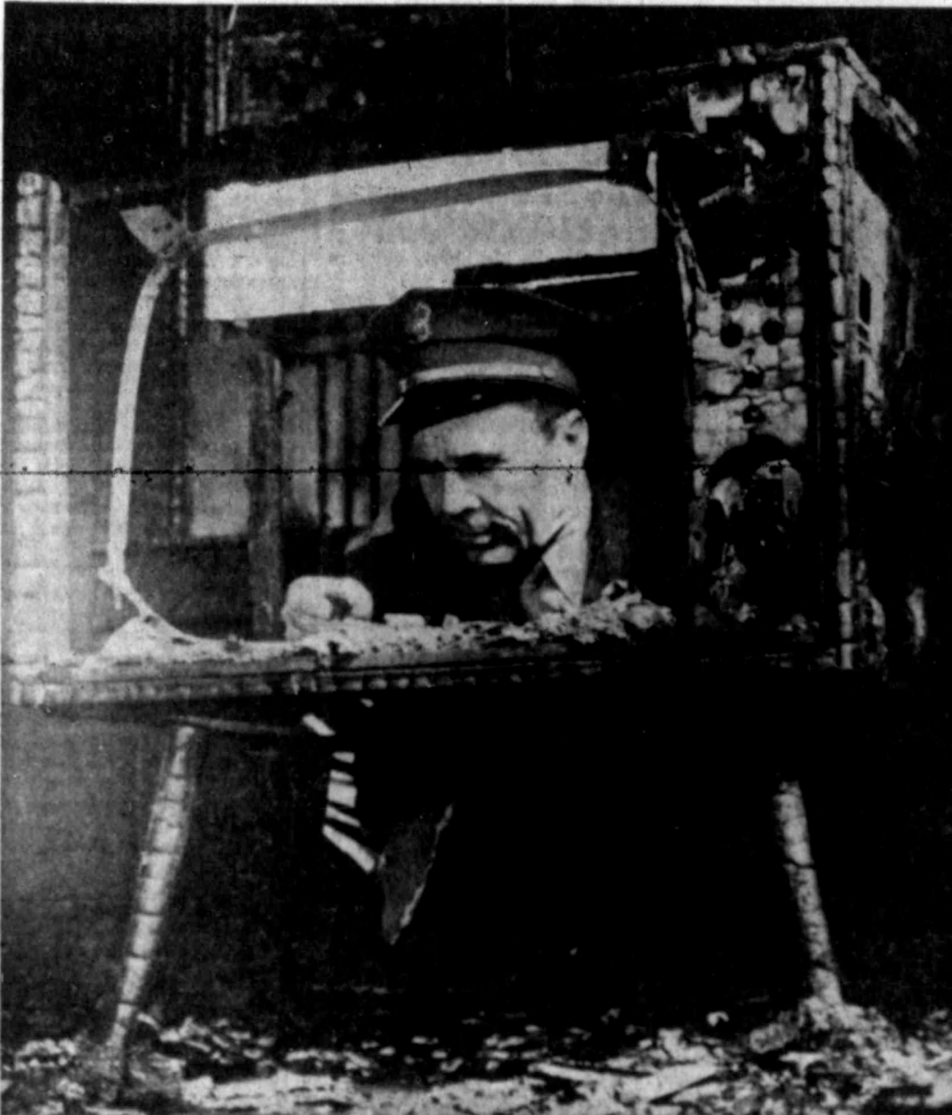
Left From The Fire
