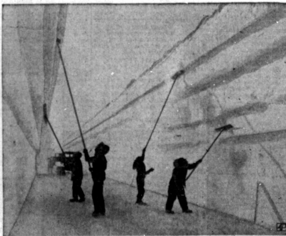
COLD HOUSEWORK —Loose snow is scraped from walls of the main tunnel at New Byrd Station in Antarctica. This is one of many housekeeping chores performed by members of the U.S. Navy's Antarctic task force in support of the scientific research program.
