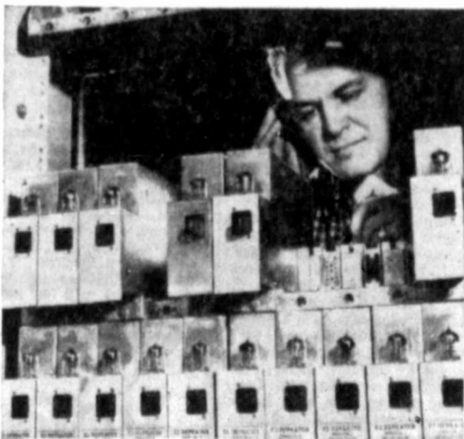
ELECTRONIC "VOICE BOOSTERS," attached to trunk lines that run between telephone central offices, keep voice volume at a strong, clear conversational level, prevent fade-out caused by distance. Latest "boosters" use Bell transistors, permit you to hear even better on your calls.
