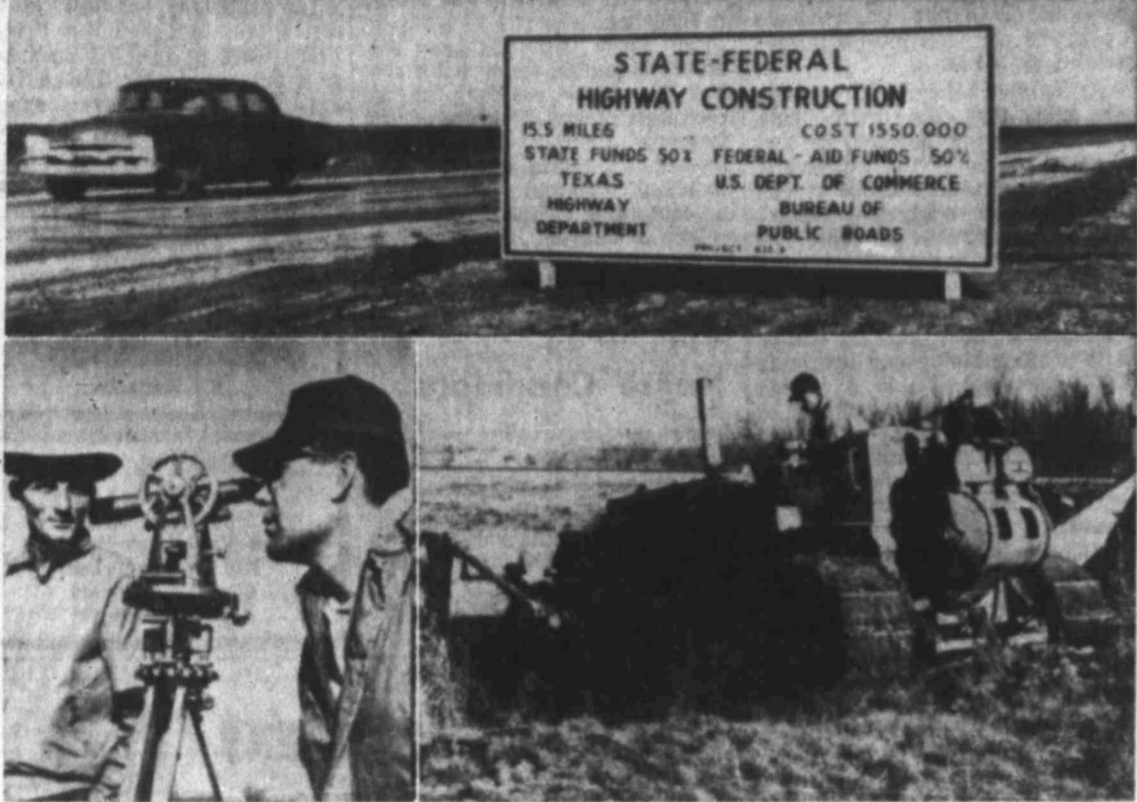
U.S. 87 Rebuilding Project Gets Under Way
