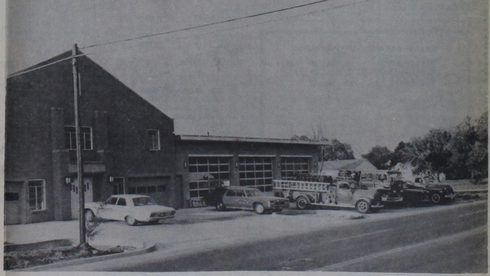
INTO THE NEW —The Dimmitt Volunteer Fire Dept. rolled its vehicles into their new garages for the first time last Thursday. During the day, Fire Marshal and Mrs. Guy Waldrop started moving into their apartment on the second floor of the new fire station. That night, the city's volunteer firemen held their first meeting in the department's
