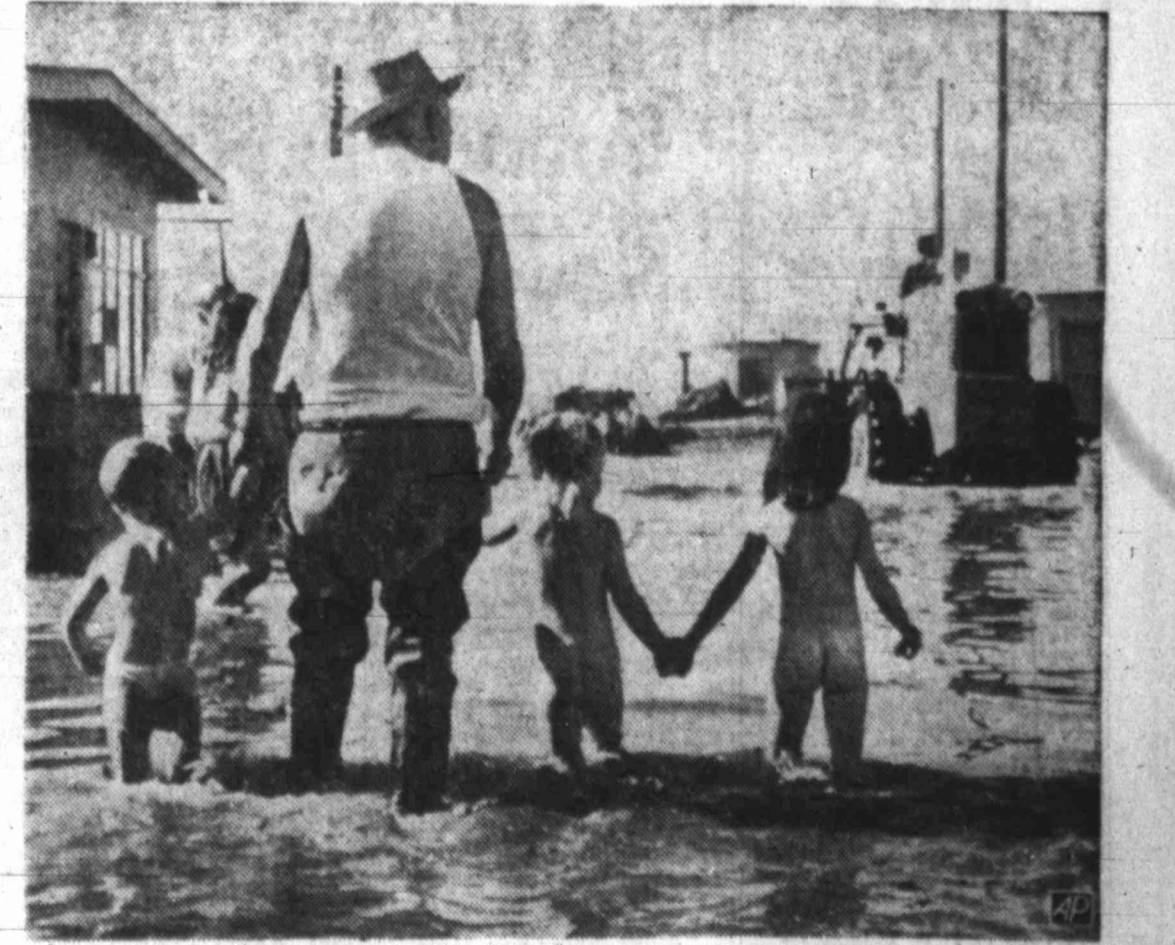
Checking Up On The Flood
