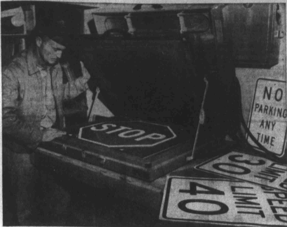
Making A 'Stop' Sign
