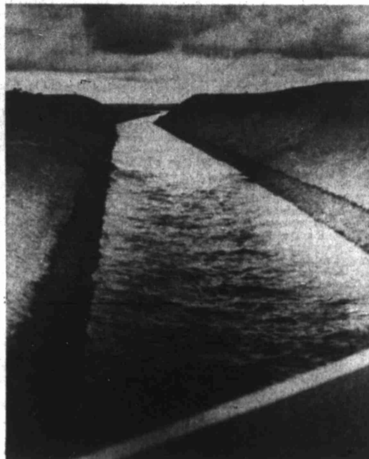
DIVERSION CHANNEL FILLED Level went up 9 feet in an hour
