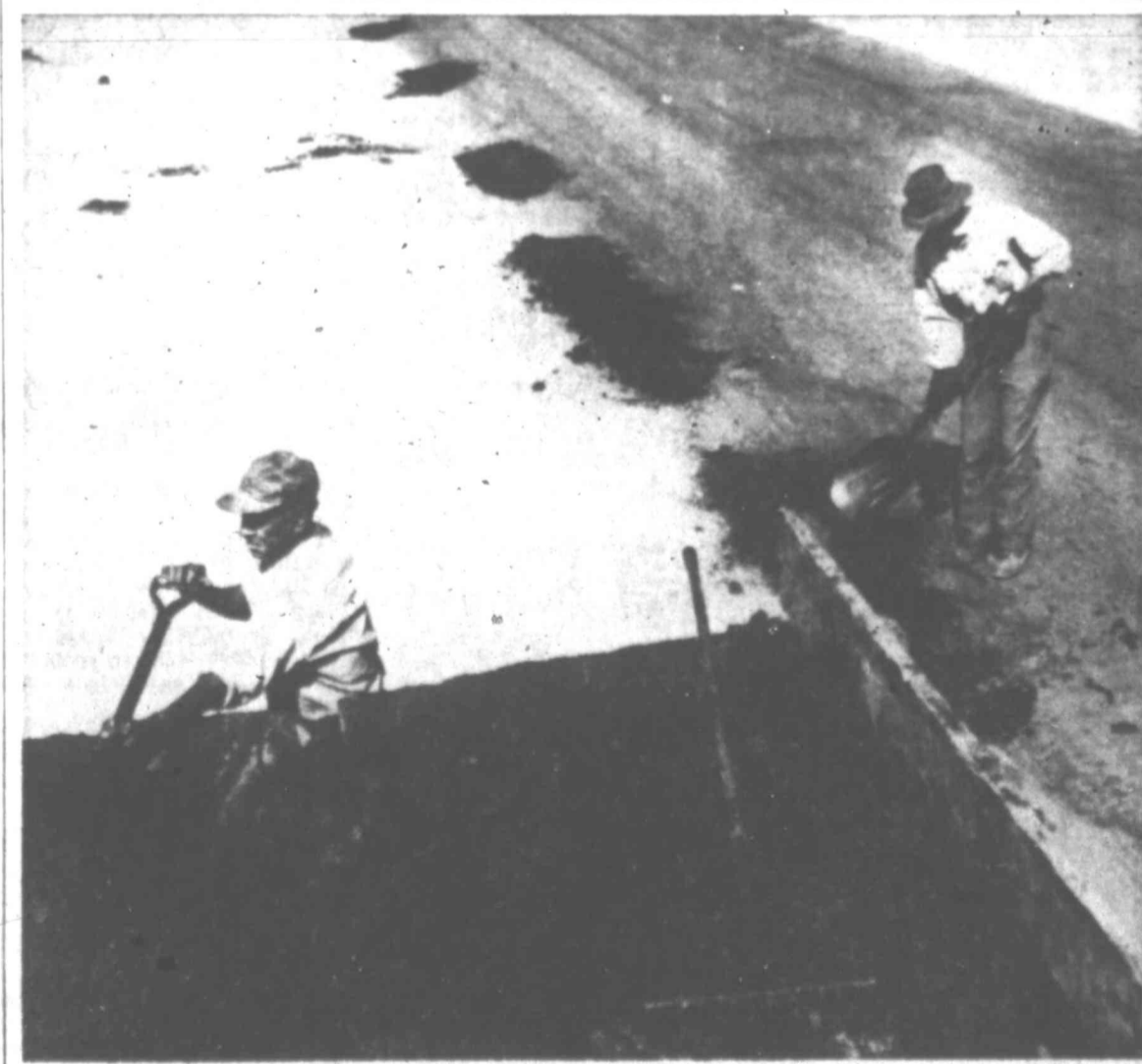
Side where streets appeared to be in a worse condition. Dirt is being hauled in to fill unpatched streets that washed out. When work on the North Side is completed, the patching crew will begin mending damaged streets in the southern portions of the city. An asphalt distributor, which will enable the city to start resurfacing streets, will probably be ready for use next week.
