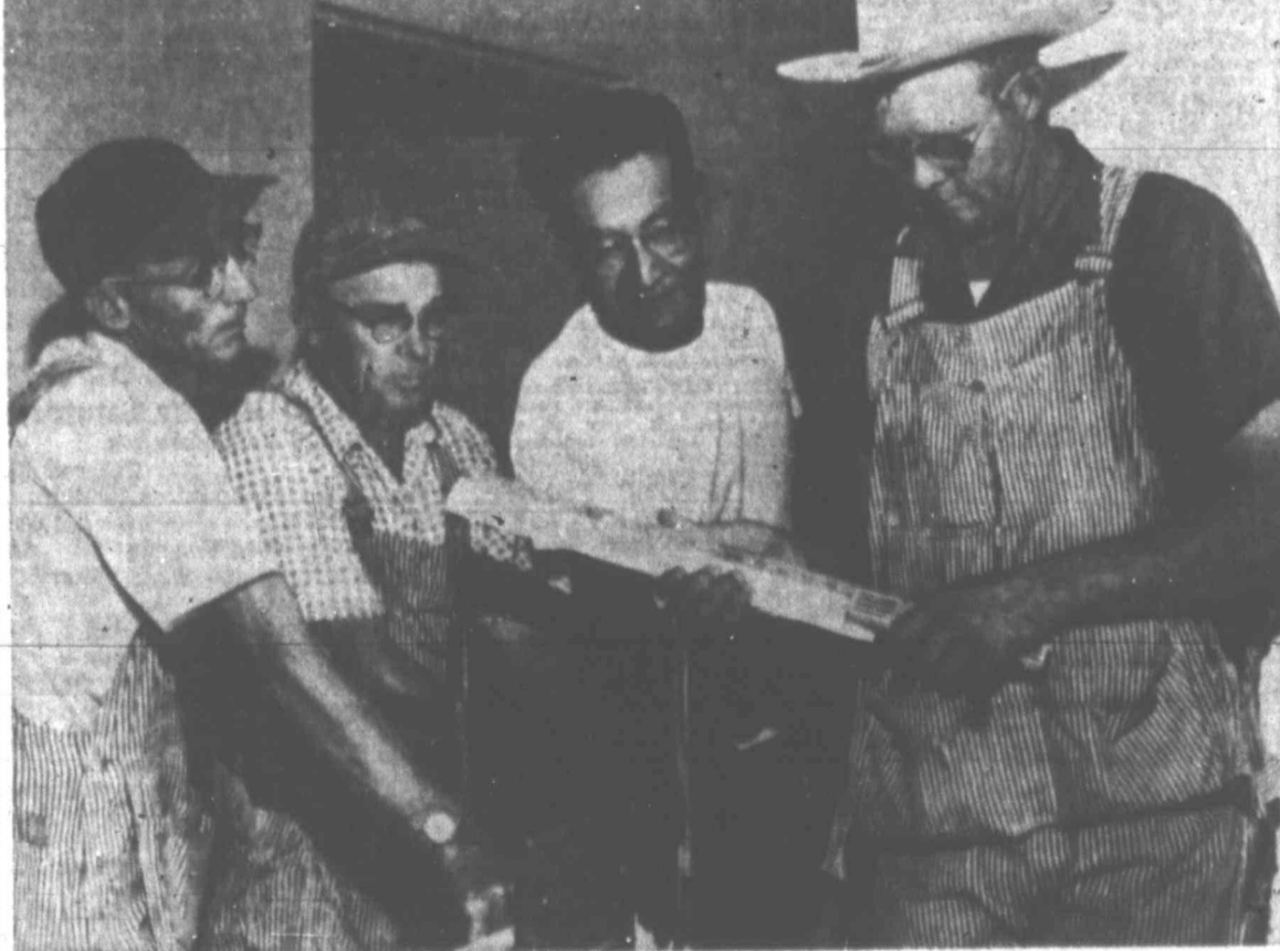
Interior trim was being installed by carpenters Fields, Nolan West, Juan Santiago and J. M. Johnson. Roy Watkins, coordinator for the labor forces, said the building is almost complete.
