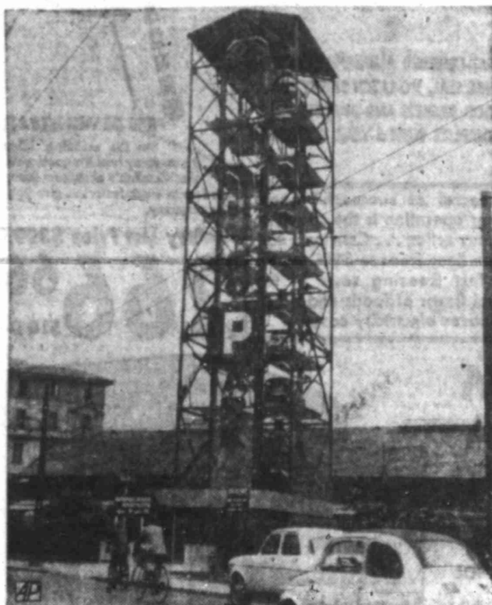
NO ROOM BELOW — This metal structure in Milan, Italy, is one solution to the parking problem. Cars driven onto elevated platform are stacked up in boxes.
