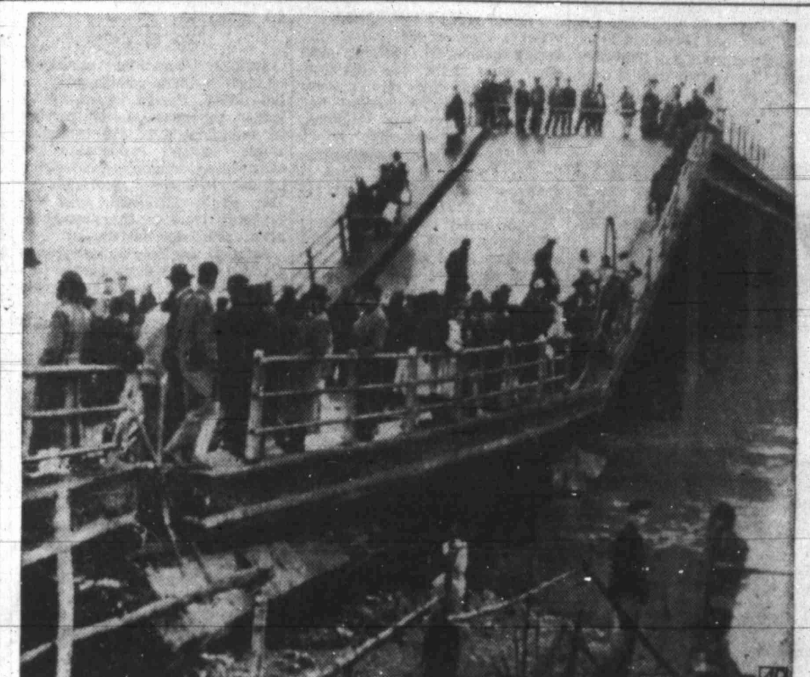
Survivors stand on part of the collapsed bridge across Chile's largest river, the Bio Bio, near Concepcion, which was wrecked during the earthquake. Two days of earthquakes followed by tidal waves have left at least 250 persons dead or missing in south and central Chile. (AP Wirephoto via radio from Lima).
