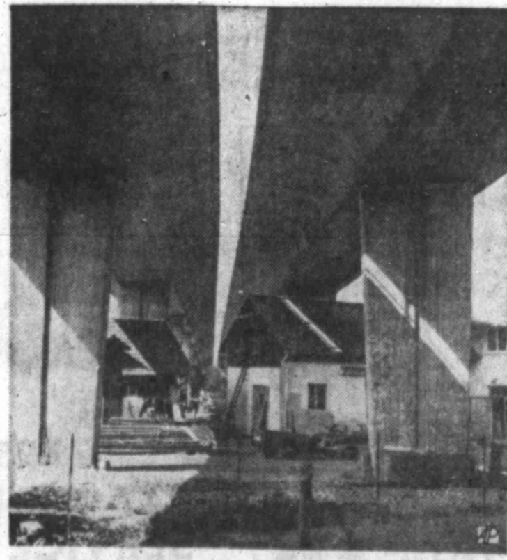
IN THE SHADE — The engineers of a dual highway in the Valley of Oos near Baden-Baden, West Germany, built the structure over the houses in its path.
